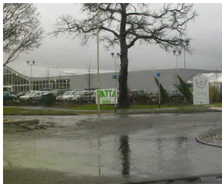
IMG014 Roundabout awash at Redfields Lane Church Crookham
