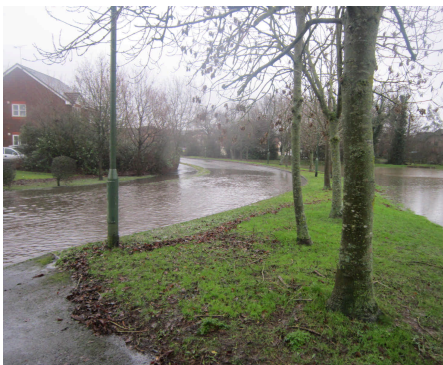
IMG013 Zebon Copse Balancing Pond overflows to roads Church Crookham
